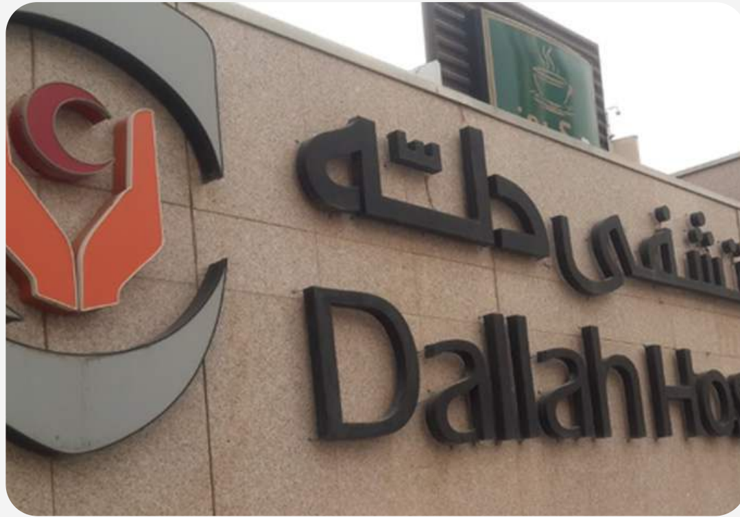
Dallah Hospital Extension
