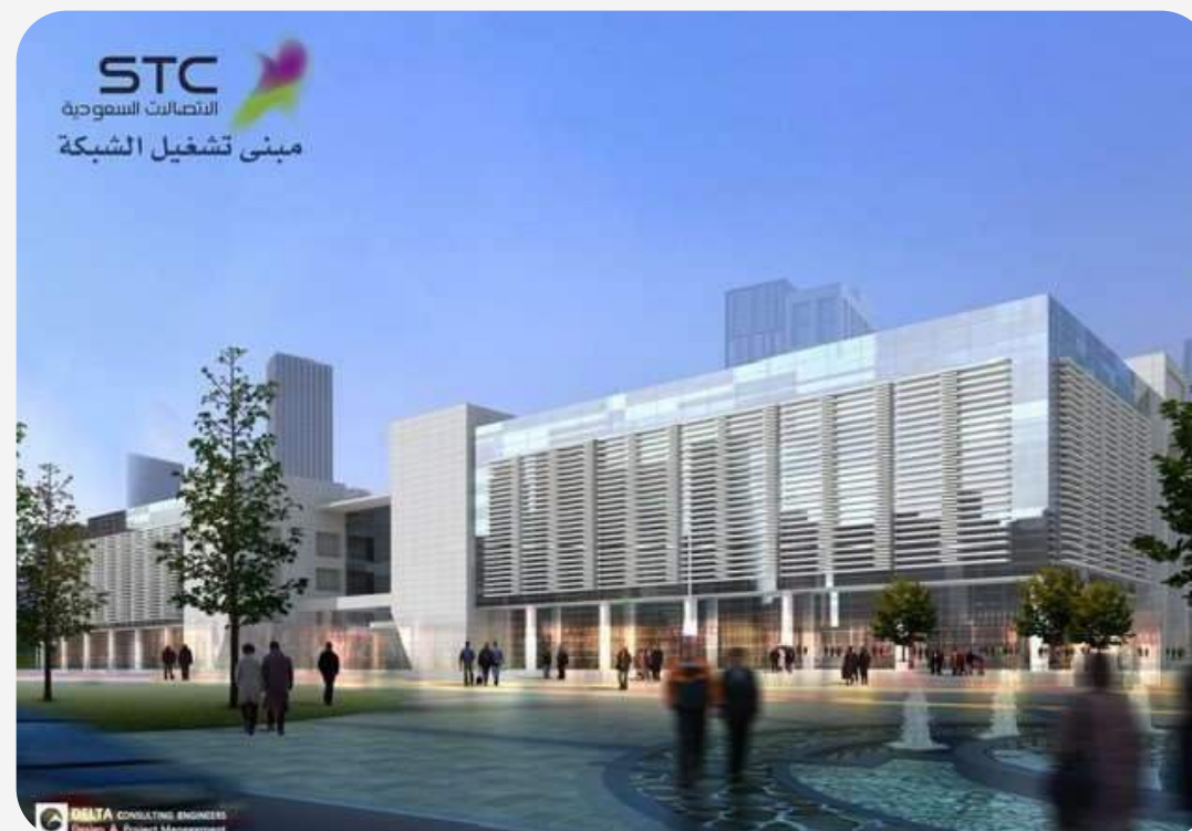
STC Building – MURSALAT – RIYADH
